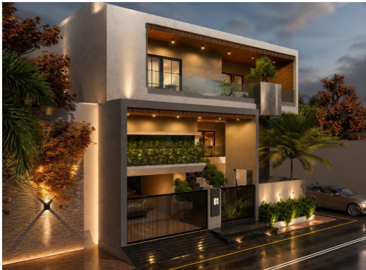
Residence elevation in stone grey and timber, dusk view
